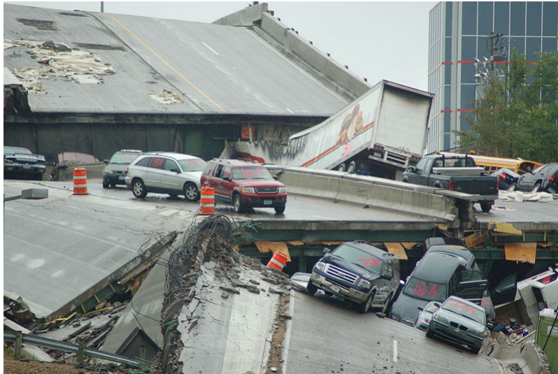
I-35W Mississippi River Bridge (2007)
